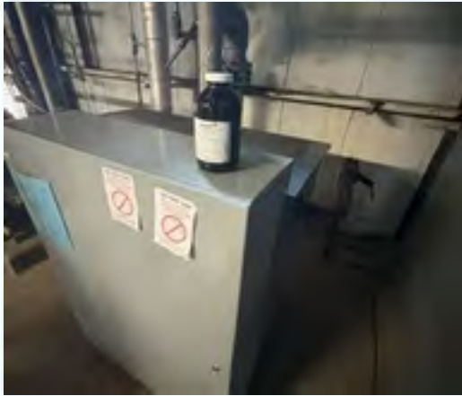
Sample 1st Floor Elevator
