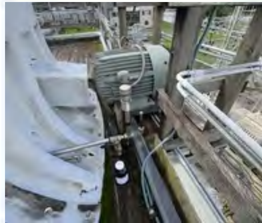
Sample Unit 14 East Gearbox
